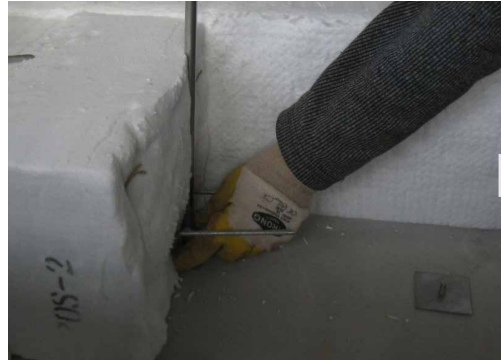
Fig. 9: Attach metallic comb-anchor
