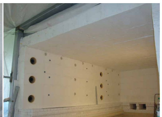
Fig. 4: After installation - industrial furnaces (with modules and bricks)
