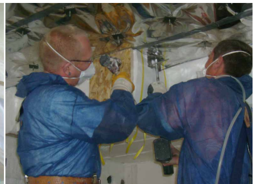
Fig. 2: Installation in the work area
