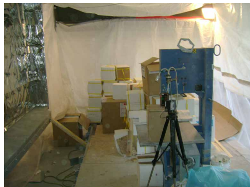
Fig. 1: Enclosed work area with filter system
