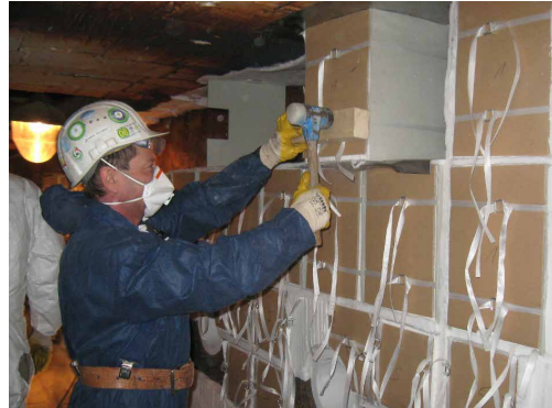
Fig. 5: Installation of prefabricated modules
