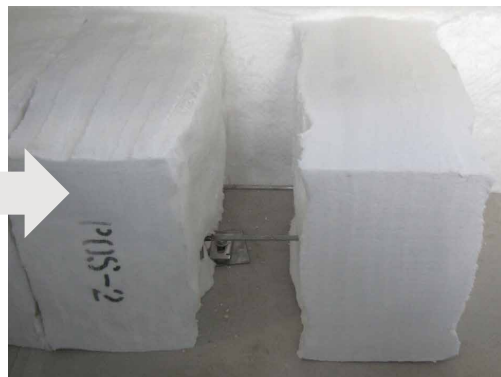
Fig. 11: Installation of the next module
