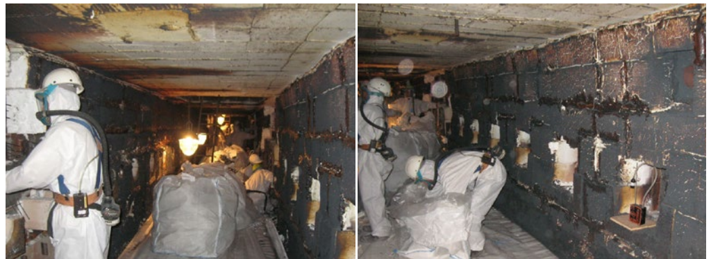
Figs. 3&4: Removed material placed into sealed plastic bags Fibrous dust reduction
