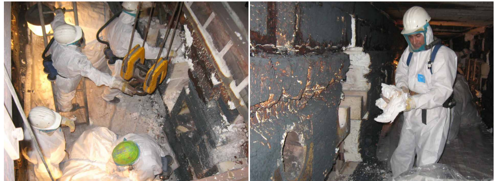
Figs. 1&2: pulling a HTIW module from the metal pins of the anchor
